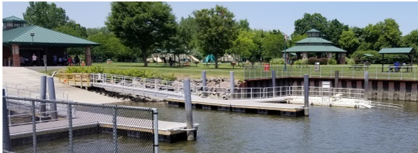
Typical Day at Haverstraw Bay Park
